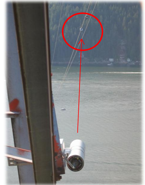
Installation of DLR Equipment
