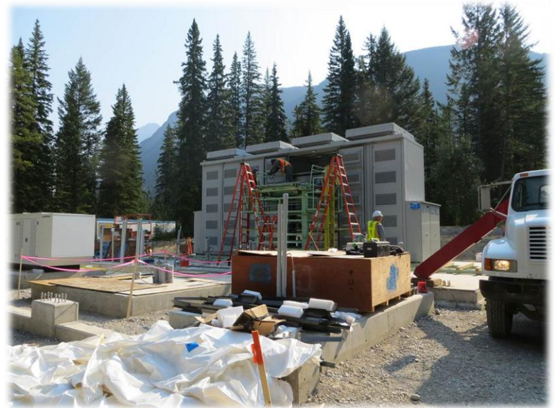
NaS Battery Installation
