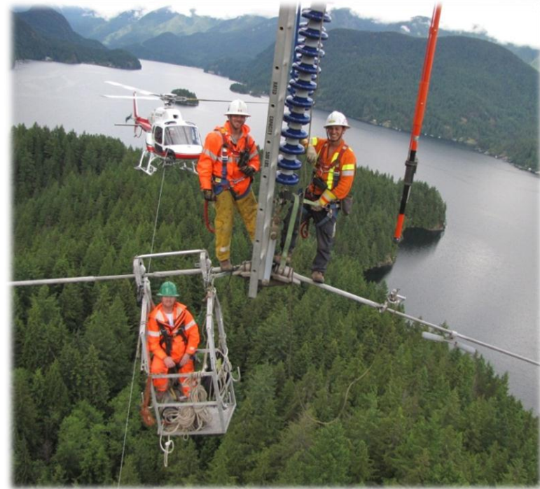
Installation of DLR Equipment
